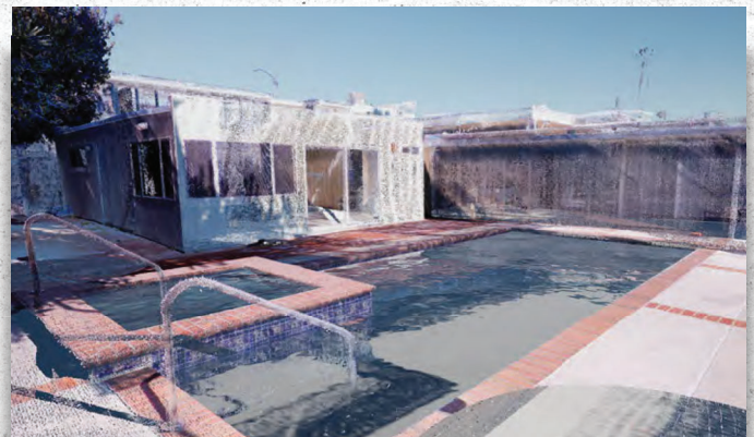
3D Laser Scan - Apartment Complex
