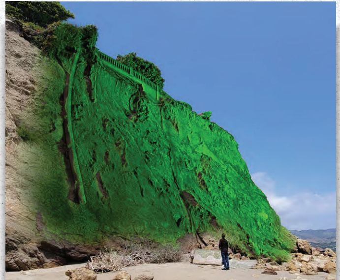
3D Laser Scan - Cliffside Erosion
